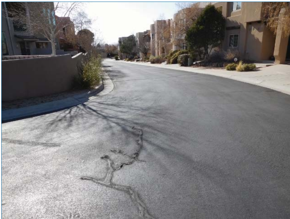
Typical street asphalt
