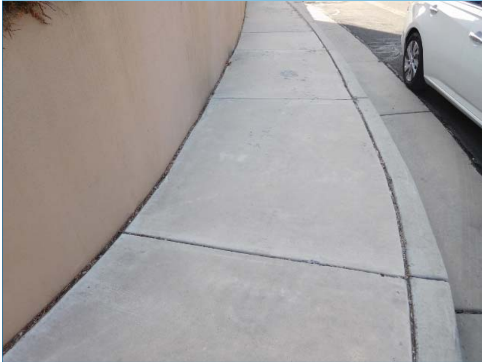
Typical concrete walkway
