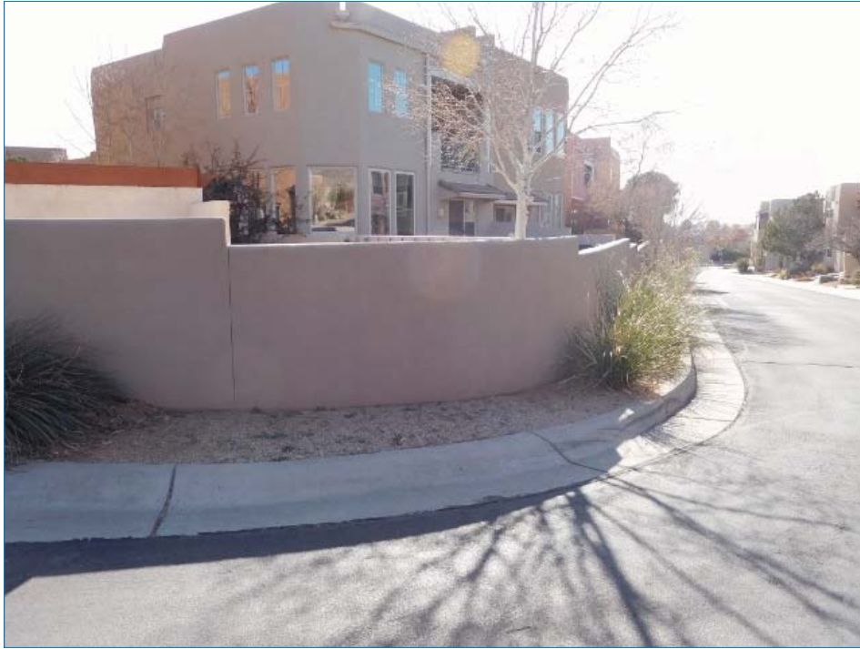
Typical stucco wall
