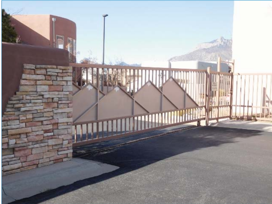
Typical vehicle gates
